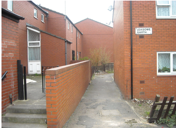
Entrance to footpath from Leasowe Garth end – criminal damage to fence next to footpath
